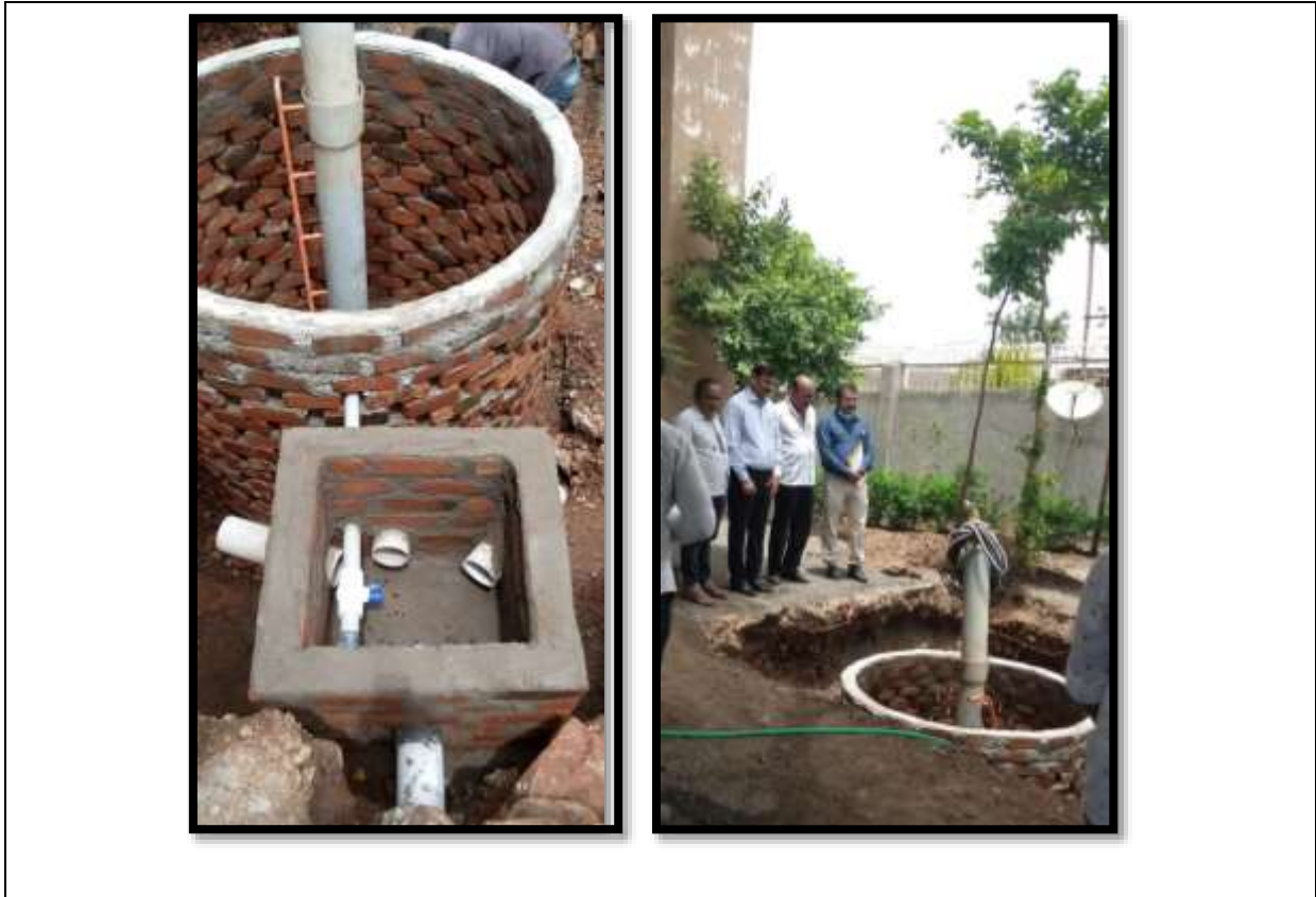
Rain Water Storage Well
