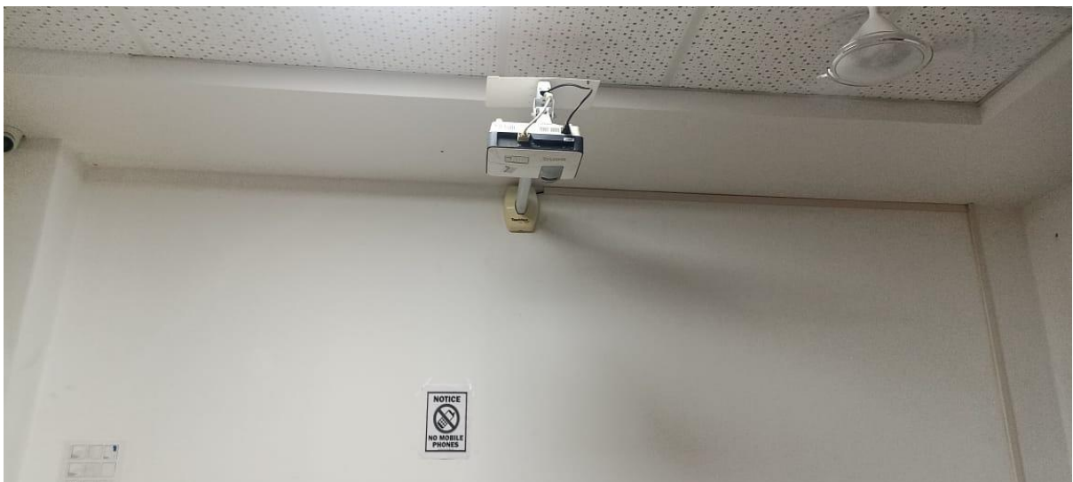
Projectors Installed at Various Points in SVM
